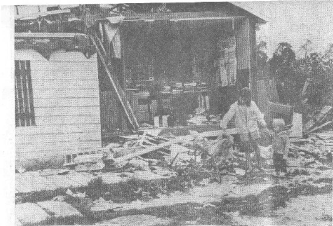
THE HORSE IS SAFE, but that discovery didn't do much to brighten the spirits of Linda and Stephen Hotal as they pushed the wreckage of their parents' Dark Lake home. The Hotal home, and those of several neighbors, were a total loss in Wednesday's storm which caused the loss of at least sixteen lives, as well as personal injury and undetermined property damage in Northern Minnesota. (MEM Photo)
